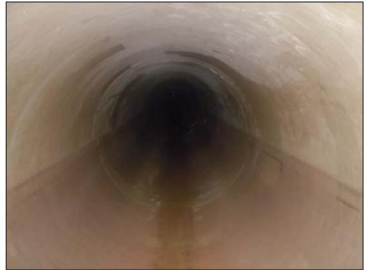
Before and After, Sewer Lining, Short Term Corrective Action Plan, Rouge Valley Sewage Disposal System ( Photos courtesy Wayne County )
